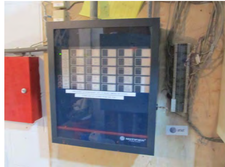
Each building has an original zone-type fire alarm control panel that has exceeded its expected useful service life
