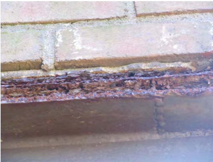
Rust damaged lintels noted at some locations
