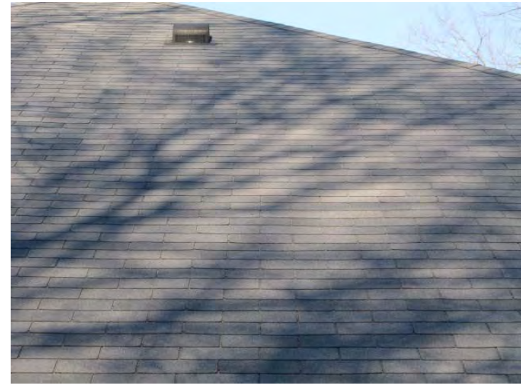
Conventional three-tab roof shingles in generally good condition
