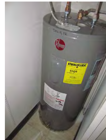
Typical unit-level electric domestic hot water tank
