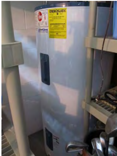
Newer domestic hot water tank that serves laundry room located at Building C
